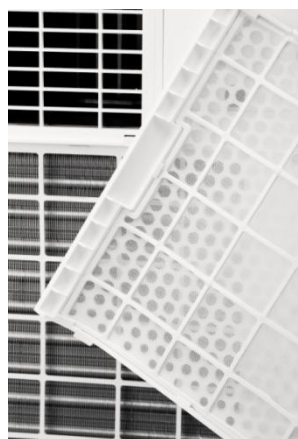
Pic1. Switch off the unit and remove the air filters.
